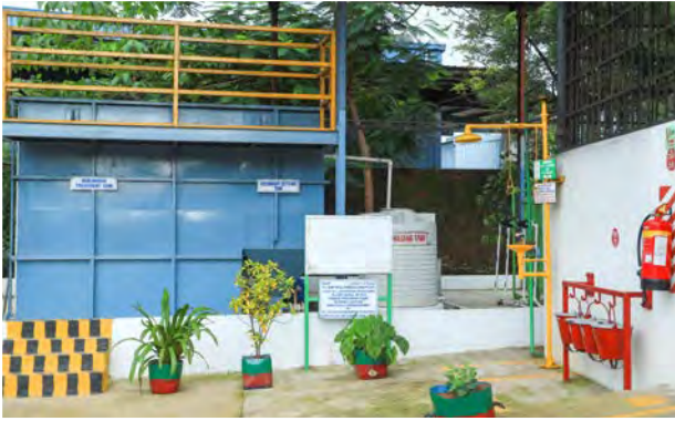
Sewage Treatment Plant
